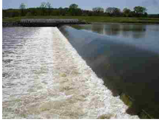
Figure 1: Typical Low-Head Dam, (NIOSH, 2010)
